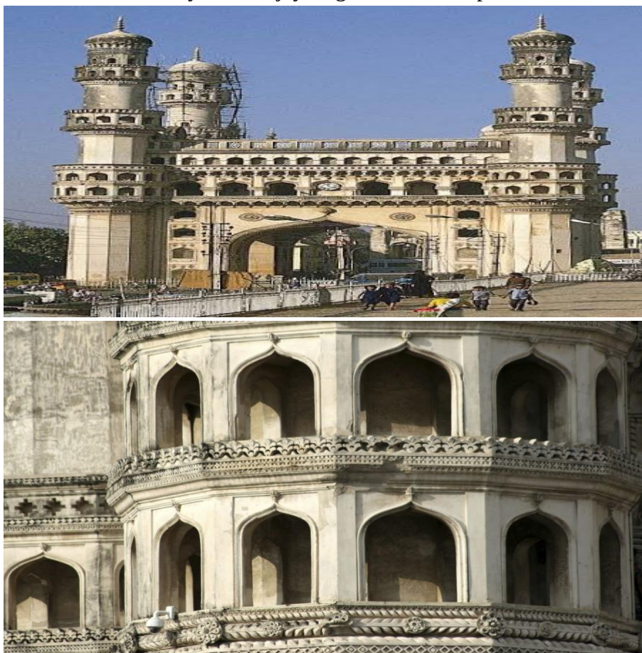
Stucco detailing on the Charminar.
